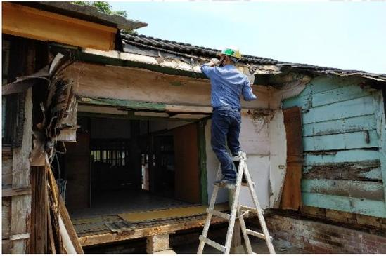
A worker on a ladder is working on the damaged roof and wall of a traditional building. The structure is in a state of disrepair, with missing tiles and crumbling plaster. |
