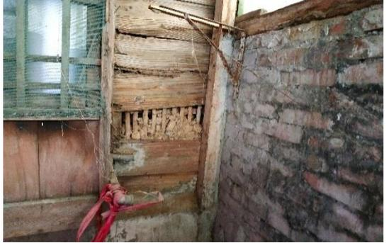
A close-up view of the damaged rainwater board in the front courtyard. The board is broken and sagging, with debris visible.                                                |
