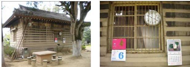
Figure9. The building for worship equipment
